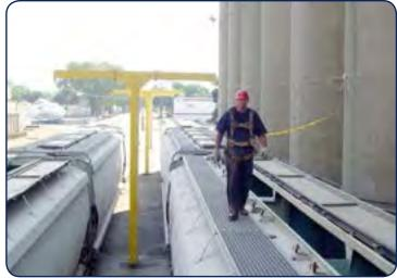
Conforms to EN 795, OSHA, ANSI, AS/ NZS standards and has been tested to meet EN 795 Class C standard.
